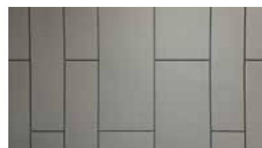
Offset joint vertical installation
