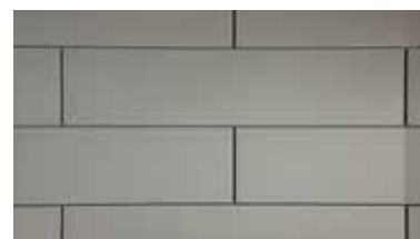
Offset joint horizontal installation
