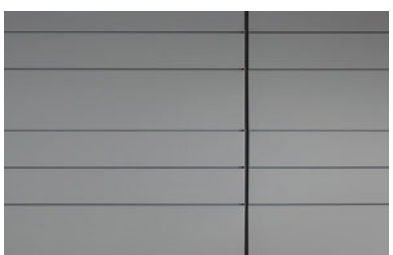
Horizontal stack installation
