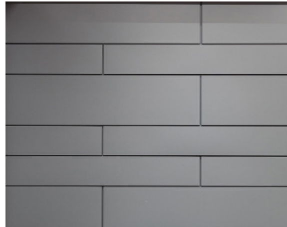
OFFSET HORIZONTAL INSTALLATION
