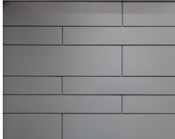
INSTALLATION HORIZONTALE INTERCALÉE
